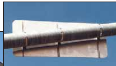
Mast Arm Sign Installation
